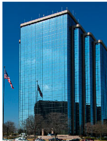
In August, Equastone bought 13 buildings in suburban Dallas, including this one in Richardson, Texas.
