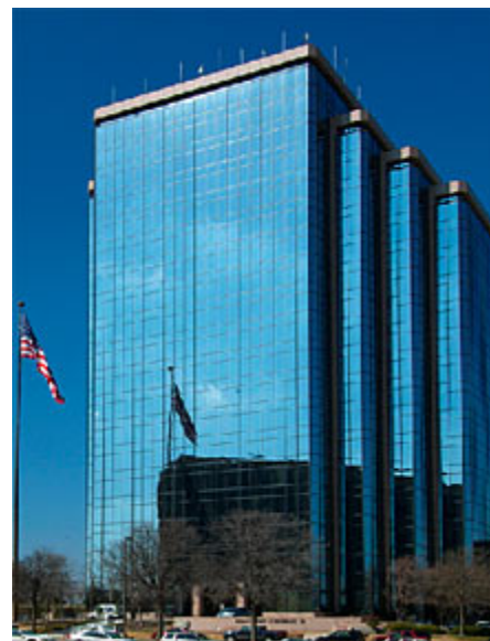
In August, Equastone bought 13 buildings in suburban Dallas, including this one in Richardson, Texas.
